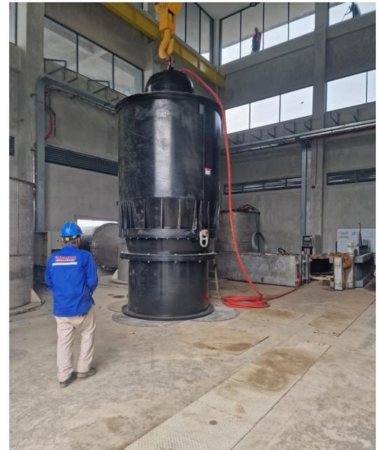
*Fig 2. Pump onsite for install*
