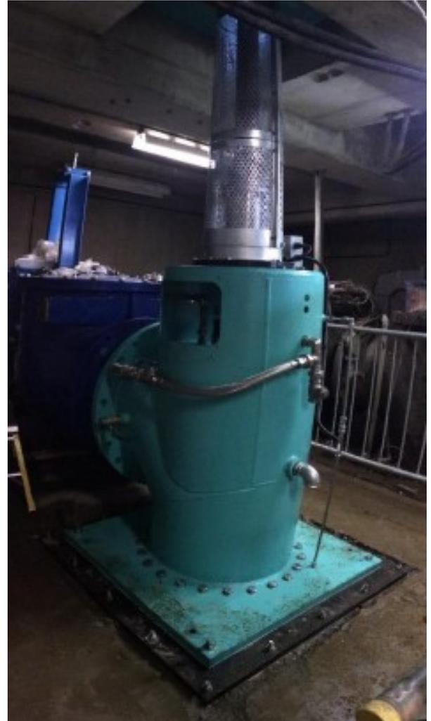
**Fig 1. Bedford Pumps suspended bowl storm pump installed at Elland Lowfield Pumping Station.**
