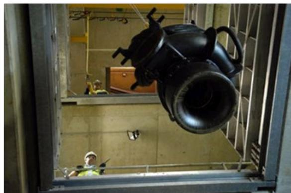
*Fig 5. Pump being lowered into the shaft*
