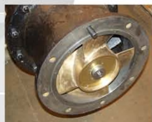
Pump fully refurbished
