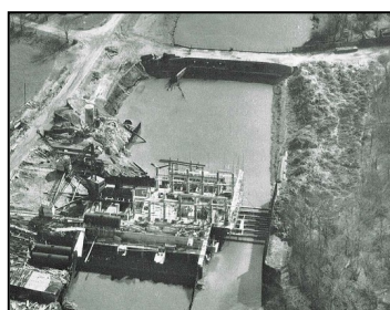
Altmouth Pumping Station constructed in 1972
