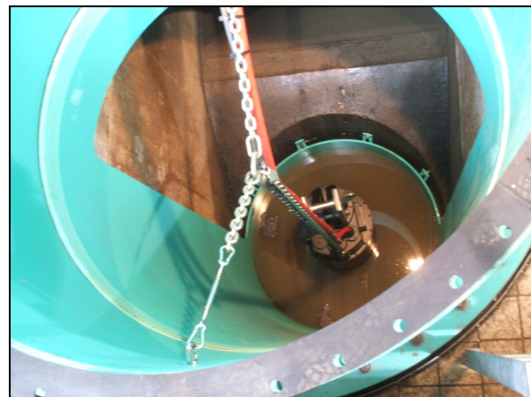
Pump installation at Altmouth Pumping Station
