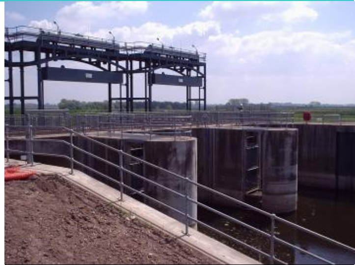
Welmore Lake Sluice
