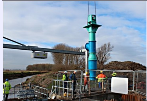
Bedford Pumps Fish Friendly pump being installed at Cam Pumping Station
