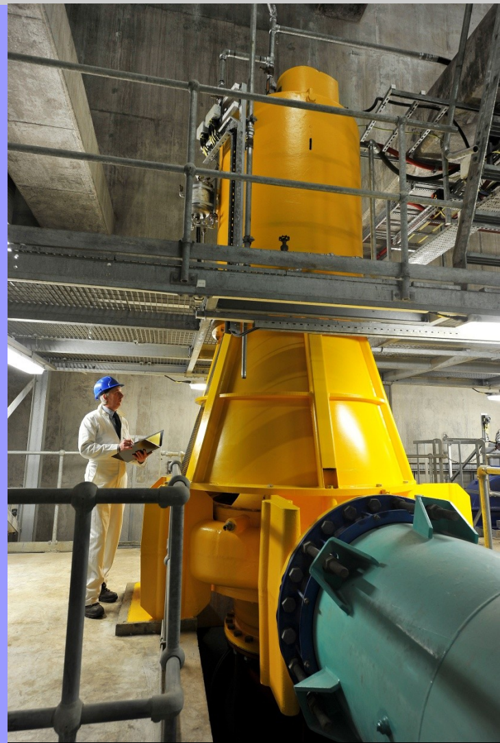
Bedford Pumps' Storm Pumps for Belfast WTW
